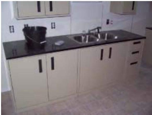
Installed cabinets in a FEMA trailer
