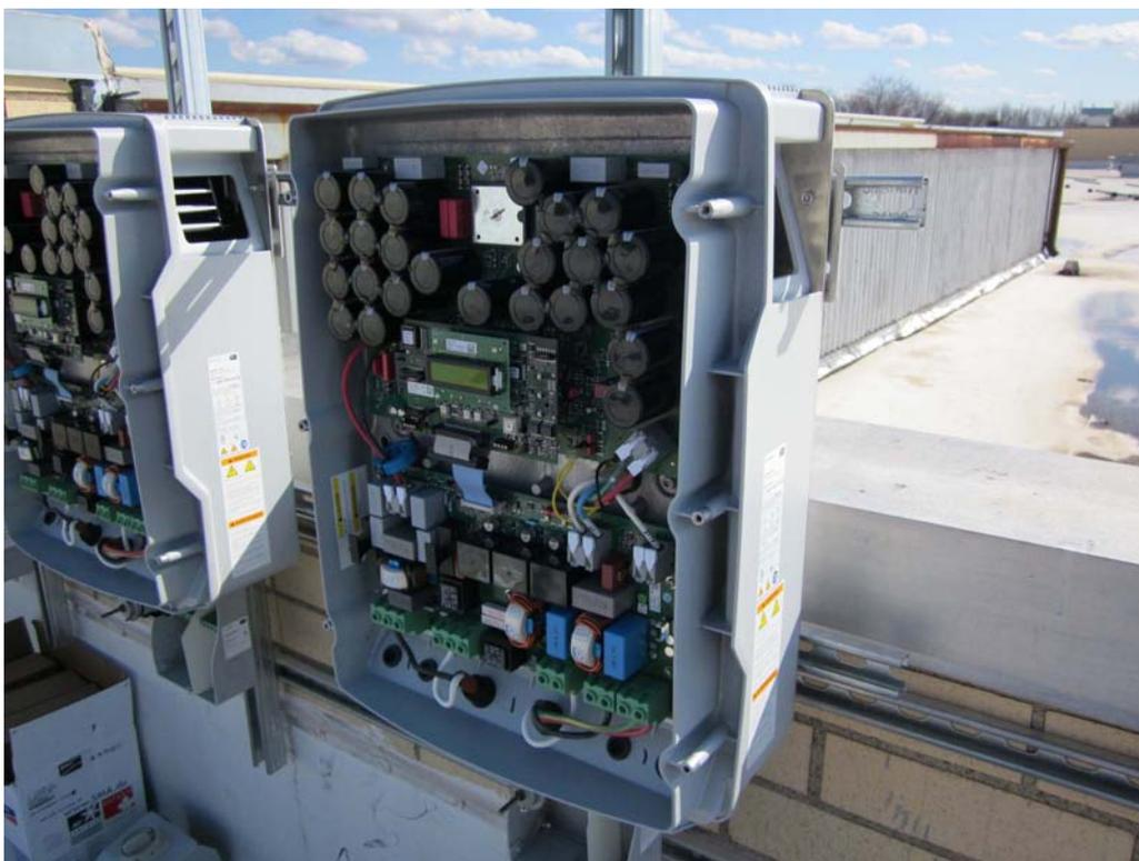
Inverters atop the roof convert the power from DC (direct current) to AC (alternating current)
